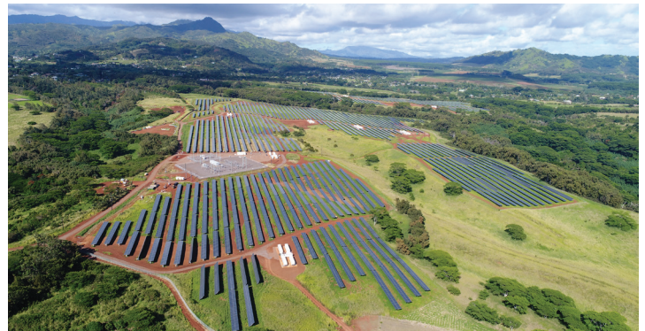
Applied Energy Service's (AES) Lawai Project. Photo courtesy: AES.
